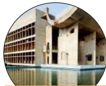
Capitol Complex Chandigarh
